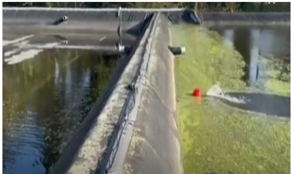
Basin – clear water after 7 days of treatment (left). Right treatment started.
